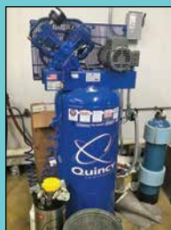
5-HP Quincy Tank Mounted Vertical Air Compressor
